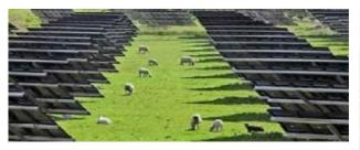
Adequate spacing between rows of panels is necessary to avoid overshadowing. Vegetation will grow between these rows and this vegetation will require management. The image to the right shows the 1.4MW Wheal Jane solar PV farm, Cornwall. Image courtesy of Lightsource Limited.
